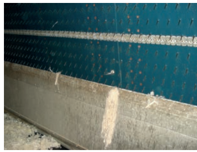
Detail of the back of the apron belts, showing splice with fasteners.
