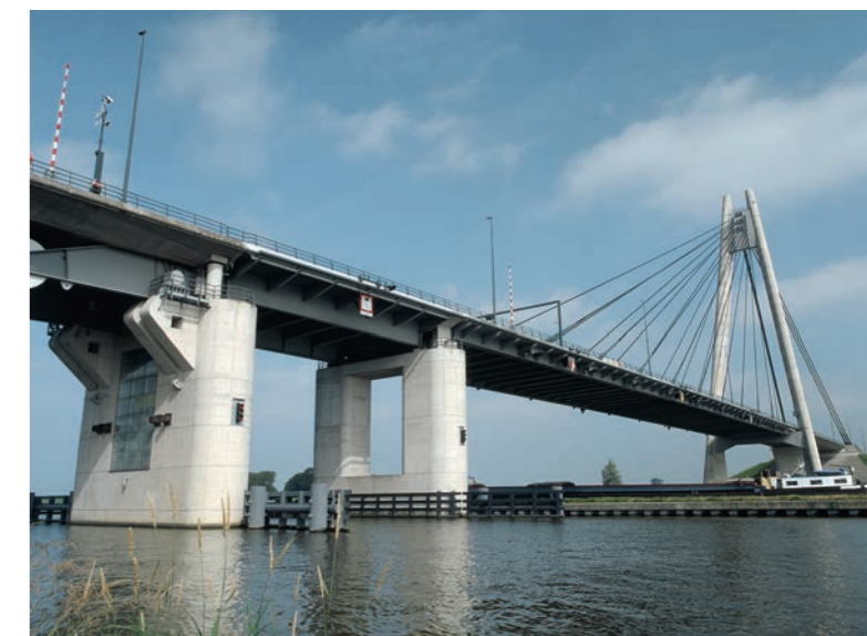
Bascule and suspension bridges
