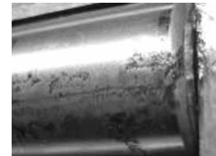
Fig. 190. Pitting on roller.
