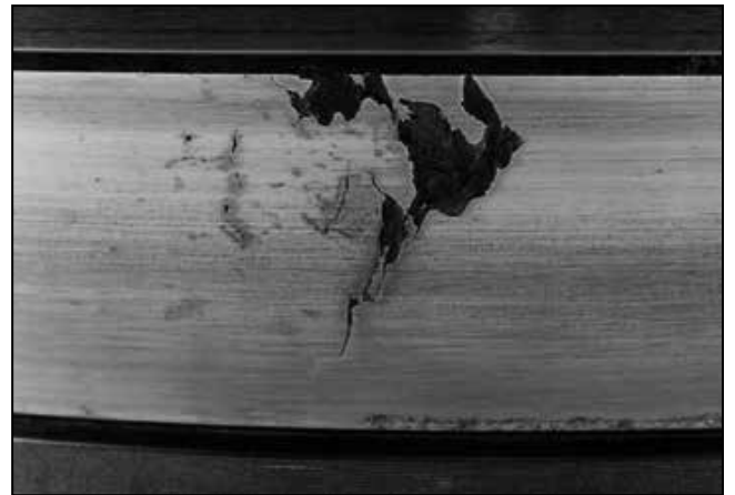
Fig. 170. Point surface origin spalling (PSO).
